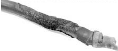
5.7 Typical battery cable problems
